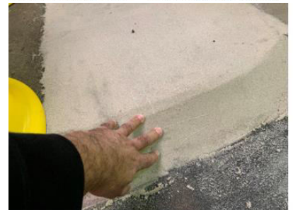
Epoxy Silica Sand Mortar for large fill
