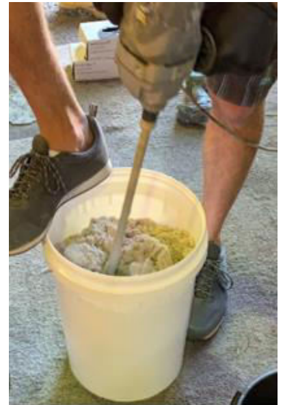
Mixing Epoxy Mortar
