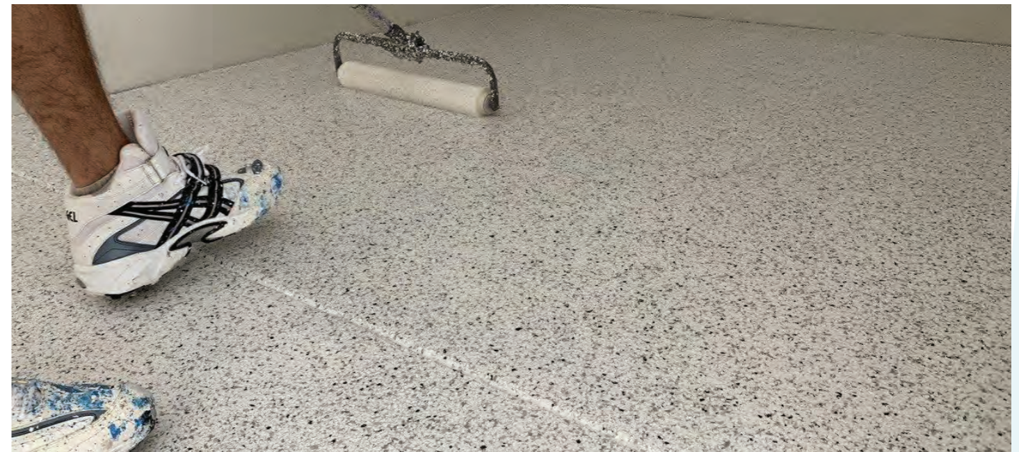
APPLYING CLEAR TOP COAT WITH A ROLLER
