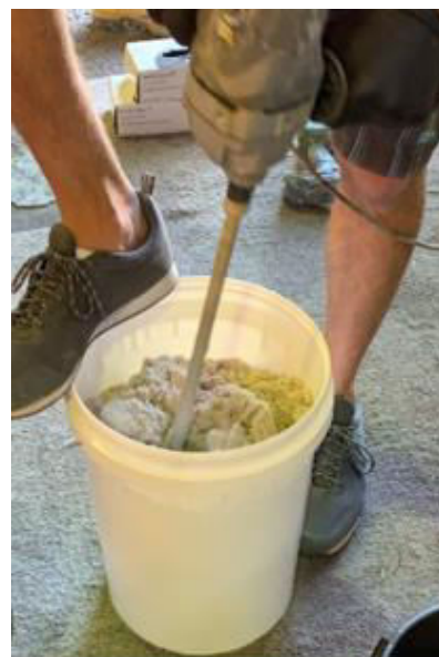
Mixing Epoxy Mortar
