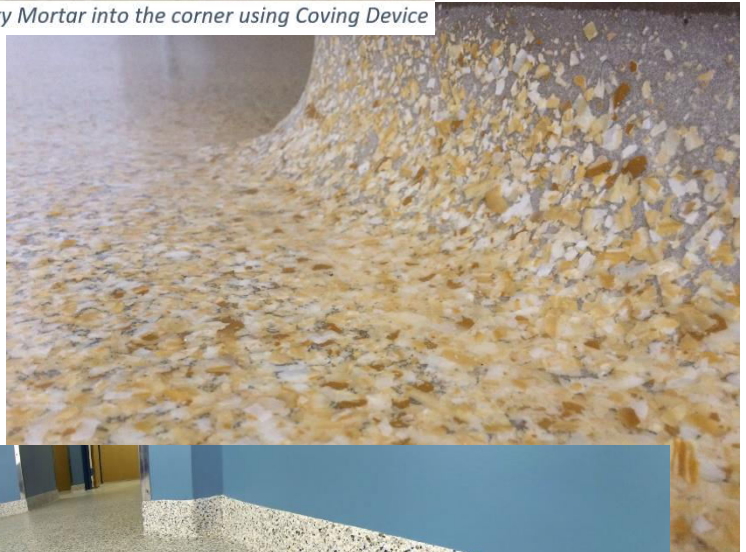
Trowelling Epoxy Mortar into the corner using Coving Device
