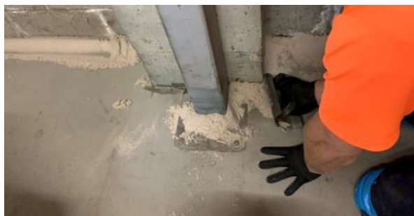
Trowelling Epoxy Mortar into the Corners
