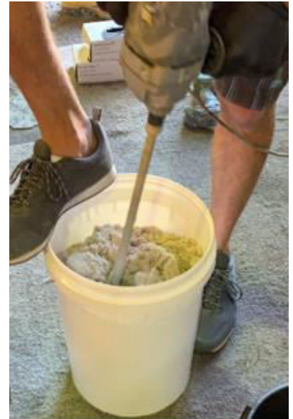
Mixing Epoxy Mortar
