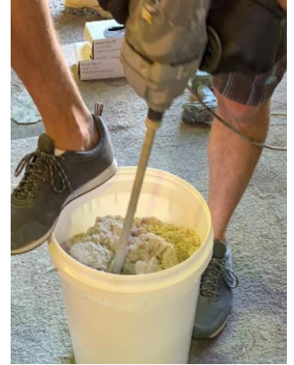
Mixing Epoxy Mortar
