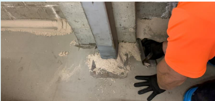
Trowelling Epoxy Mortar into the corner using Coving Device
