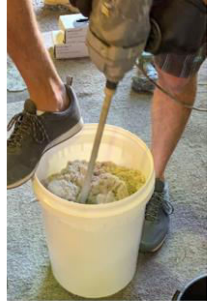
Mixing Epoxy Mortar
