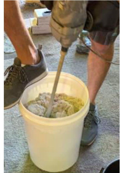
Mixing Epoxy Mortar
