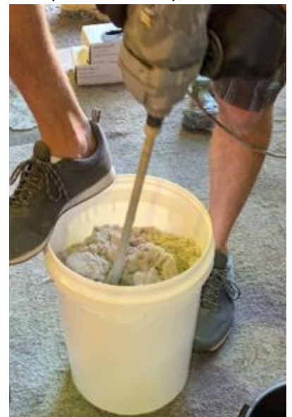
Mixing Epoxy Mortar
