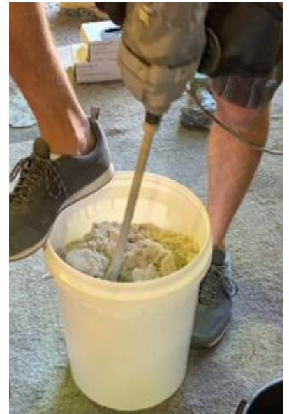
Mixing Epoxy Mortar
