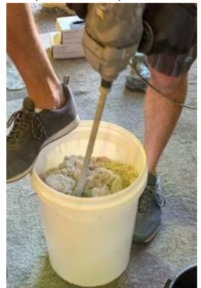
Mixing Epoxy Mortar
